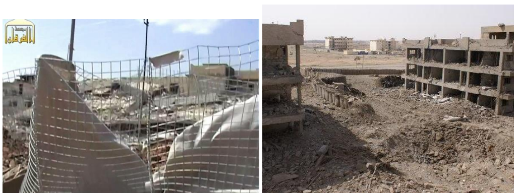
18. figure: Failed HESCO bastion (left) and standing RC structure after SVBIED attack (right)
