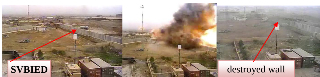
17. figure: Failure of T-Wall protection wall due to SVBIED attack
