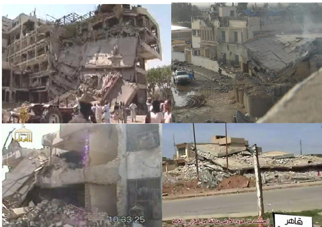
14. figure: Buildings after progressive collapse
